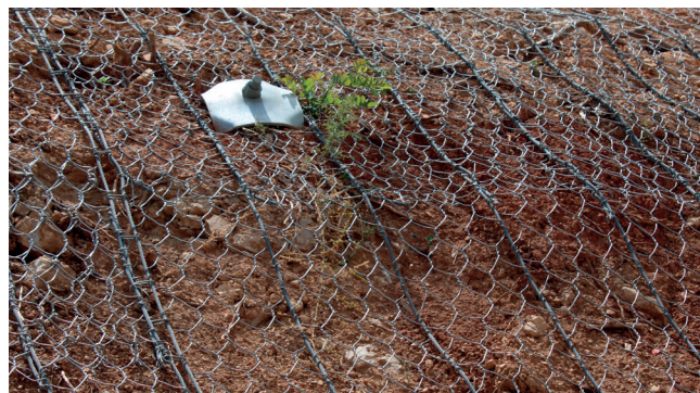
Figur 2. Steelgrid X installert i en skråning.
