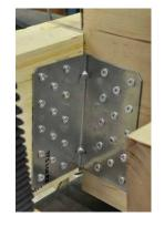
$\bullet \qquad \text{K}_{\text{ser}} \text{ according to EN 1995-1-1 for timber-to-timber joint screws* C24/GL24h} \\$
