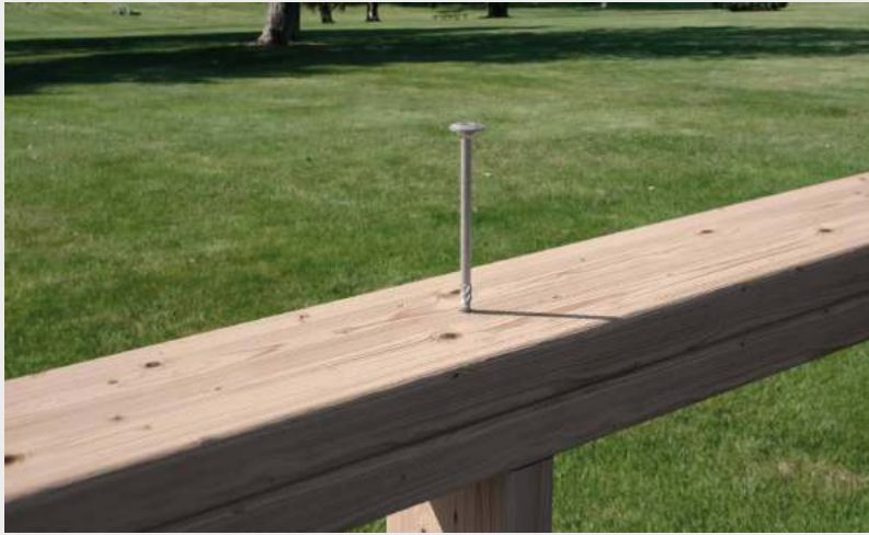
Fastening Wood Trusses outdoors.
