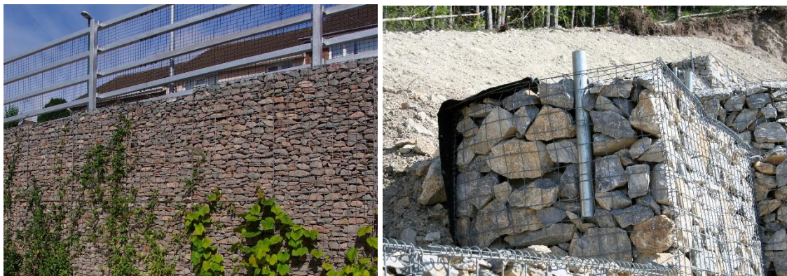
Fig. 35 – Post supporting a safety barrier within a gabions structure
